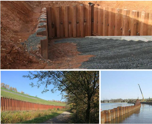
Fig. 2. Typical applications of sheet piling structures. In urban construction, they form retaining walls allowing for pre-foundation excavation (top) [14]. They provide slope stabilization in steep or uneven terrain (bottom left) [15]. In ecological applications, they are used for purposes like shoreline fortification (bottom right) [16].
